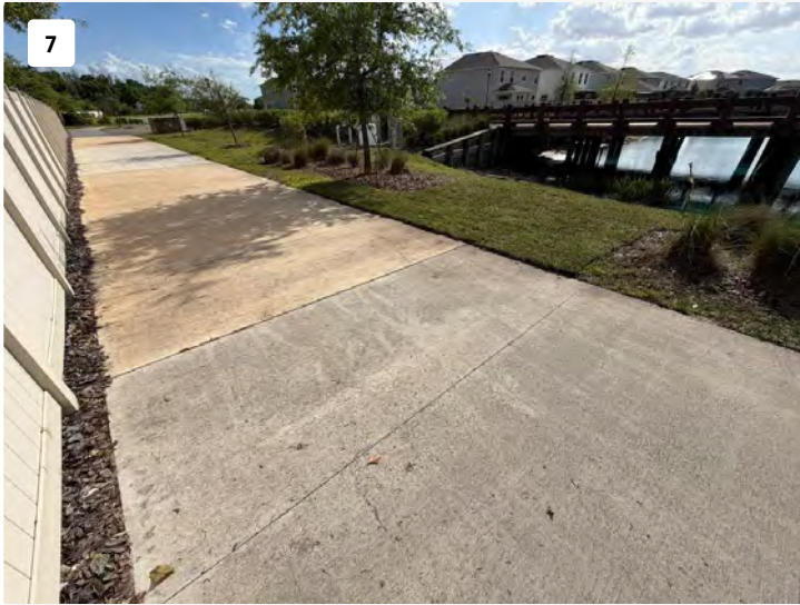
Sidewalk brushed clean after work was completed.
