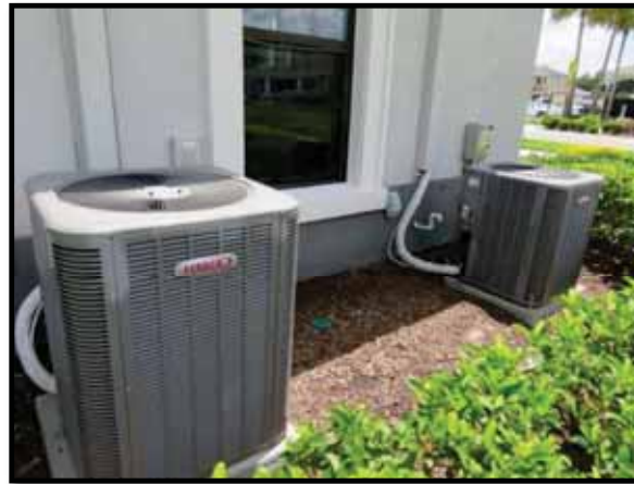
Figure 1 – HVAC Condensers
