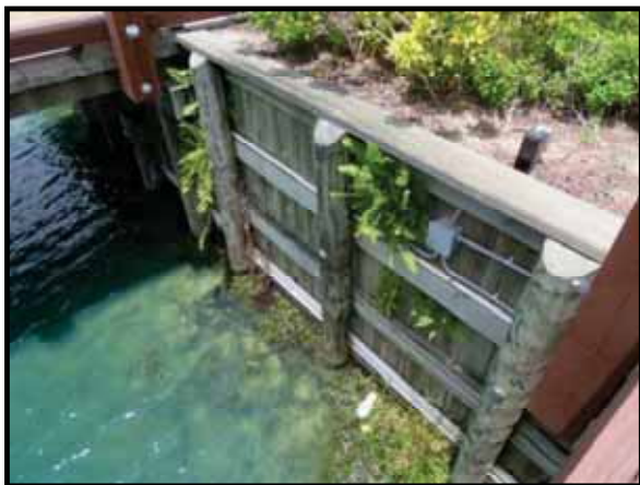
Figure 1 – Wood Bulkhead Retaining Wall
