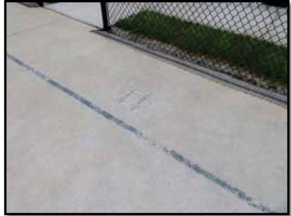
Figure 2 – Exposed Reinforcing
