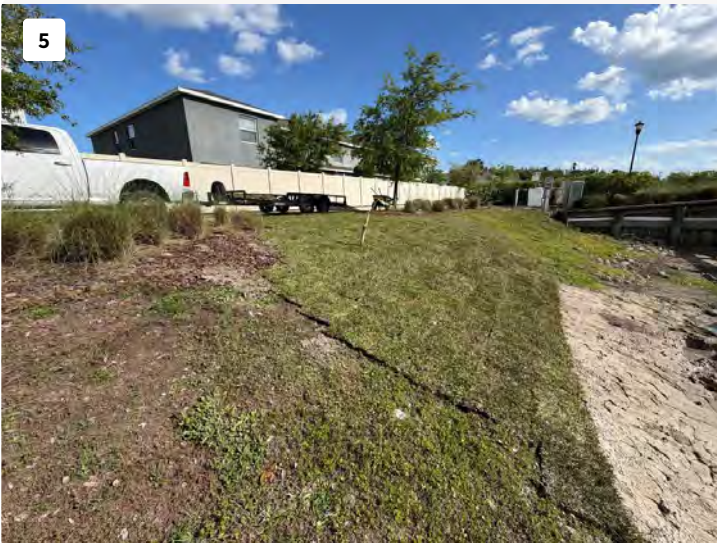
Bank graded to proper 4:1 slope, recommended by SWFWMD.
