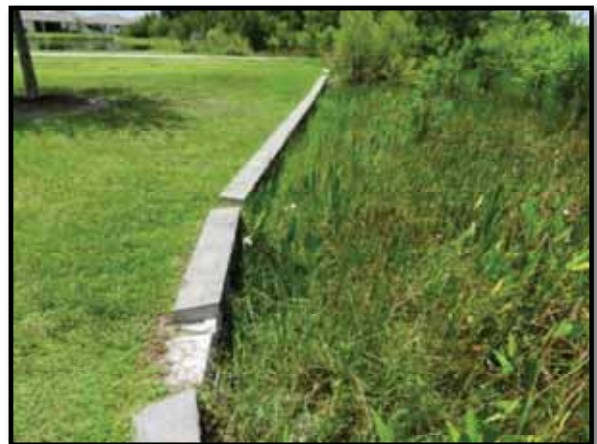
Figure 2 – Masonry Retaining Wall
